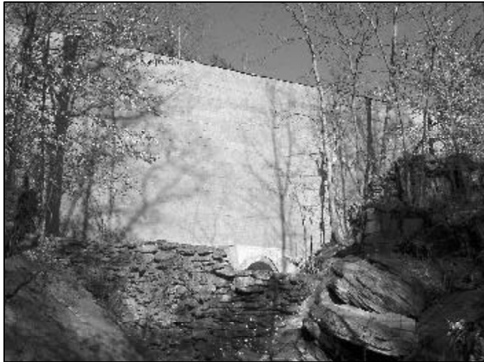
Land bridge under construction. Finished wall will be approximately 20 meters high.
